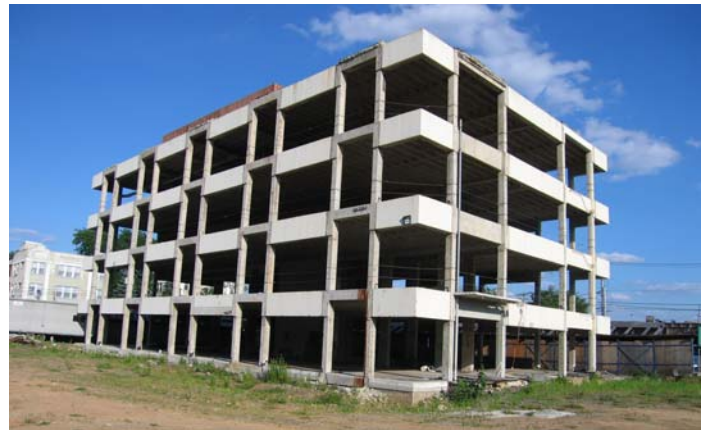
Existing Concrete Structure
